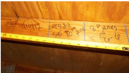
Example of Nail Spacing
